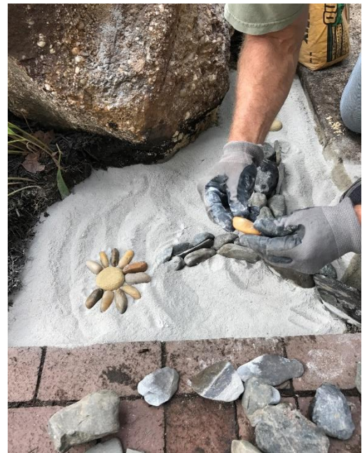
PHOTO.2 – Bob laying the stone as directed by Tim.
